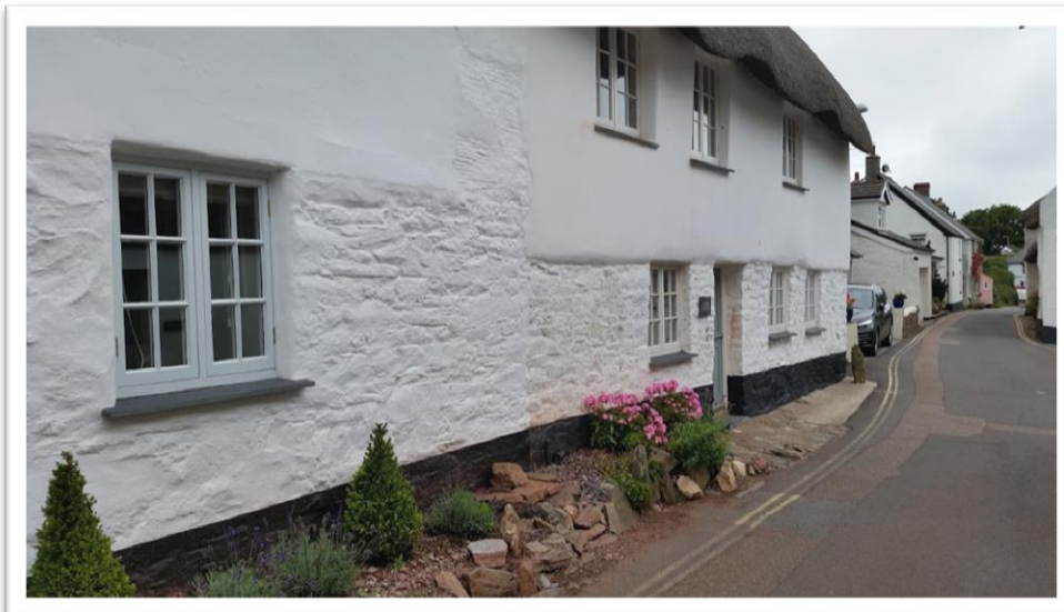
MOONRAKERS AND DYERS COTTAGE, MALBOROUGH LOWER TOWN, Malborough, South Hams, Devon
