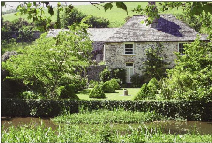
Riversbridge - a listed building
